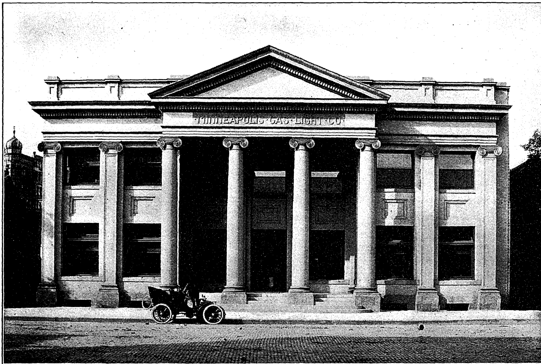
THE MINNEAPOLIS GAS LIGHT COMPANY'S BUILDING
