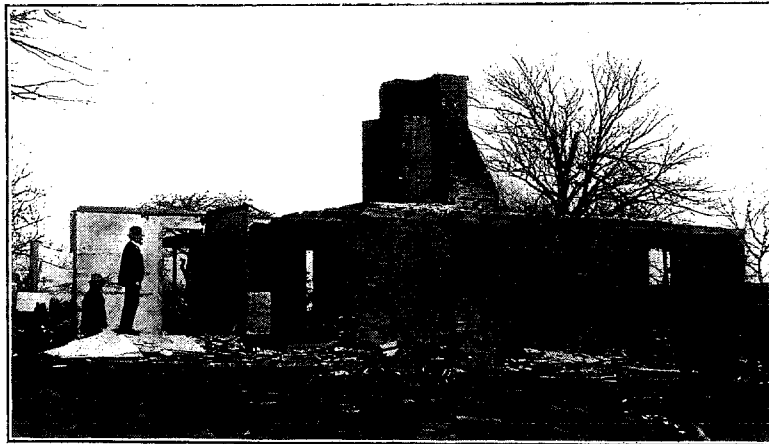
BRICK WALLS OF BENJAMIN CLAPP HOUSE.
